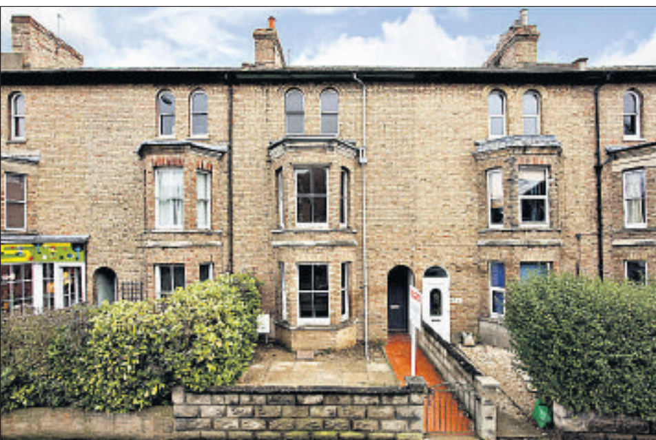
Victorian villa: The three-storey house in Iffley Road, with its bathroom, below
